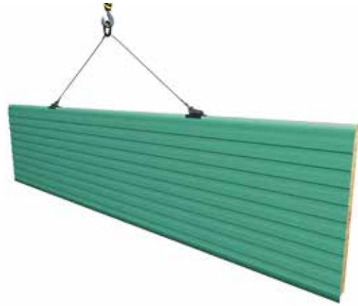
Fig. 57.: Manipulation with an RH panel on a horizontal lay-down. ("Iron" – a clamp in the panel's lock – always 2 pieces at least)
